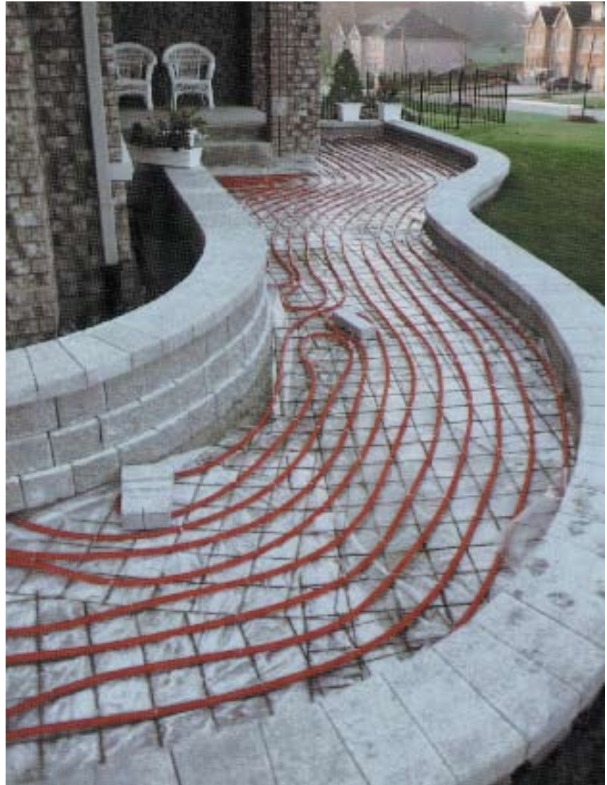
This REHAU SIM system, installed under a residential walkway which continues onto the driveway, frees the homeowner from snow removal chores and enhances safety throughout the cold season.
